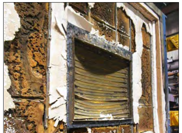
Remains of a drywall partition after a fire test The two 15mm thick layers of plasterboard have been completely destroyed by the ferocity of the fire and the fire damper blade pack itself has been completely deformed.
