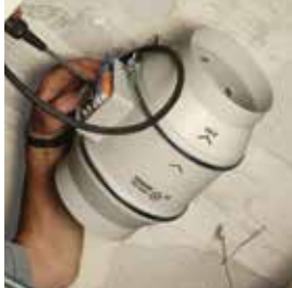
Carry out the wiring connections.
